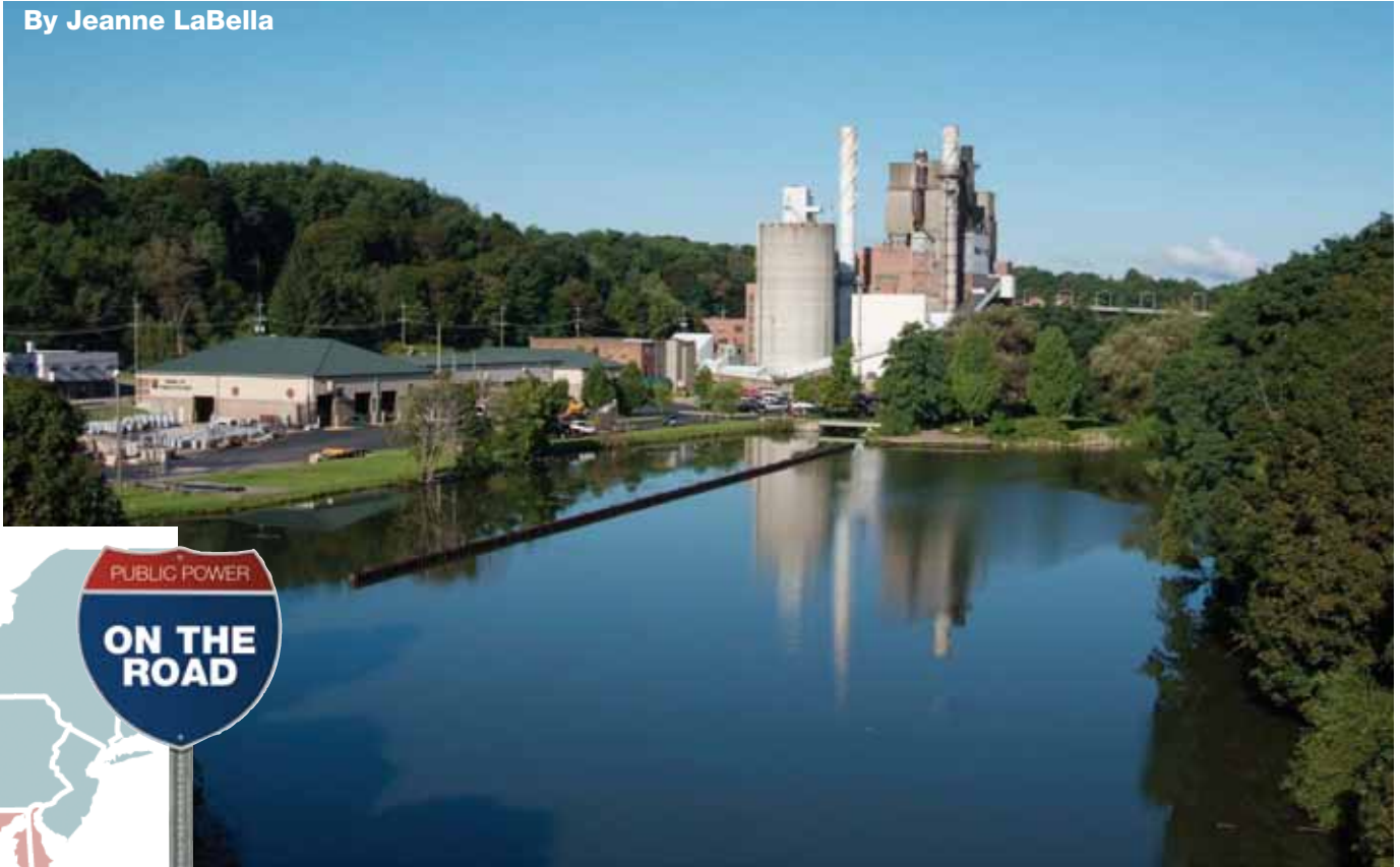
Jamestown's Samuel A. Carlson Electric Generating Station and the Board of Public Utilities Operations Center sit on the banks of the Chadakoin River.
