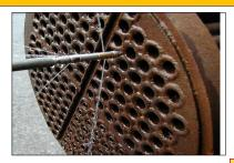
your heat exchanger is returning water to the Power Plant at or above 190 degrees Fahrenheit, you probably have calcium in your heat exchanger. The calcium can clog your heat exchanger, preventing enough of the hot water to enter your system to heat your building.
