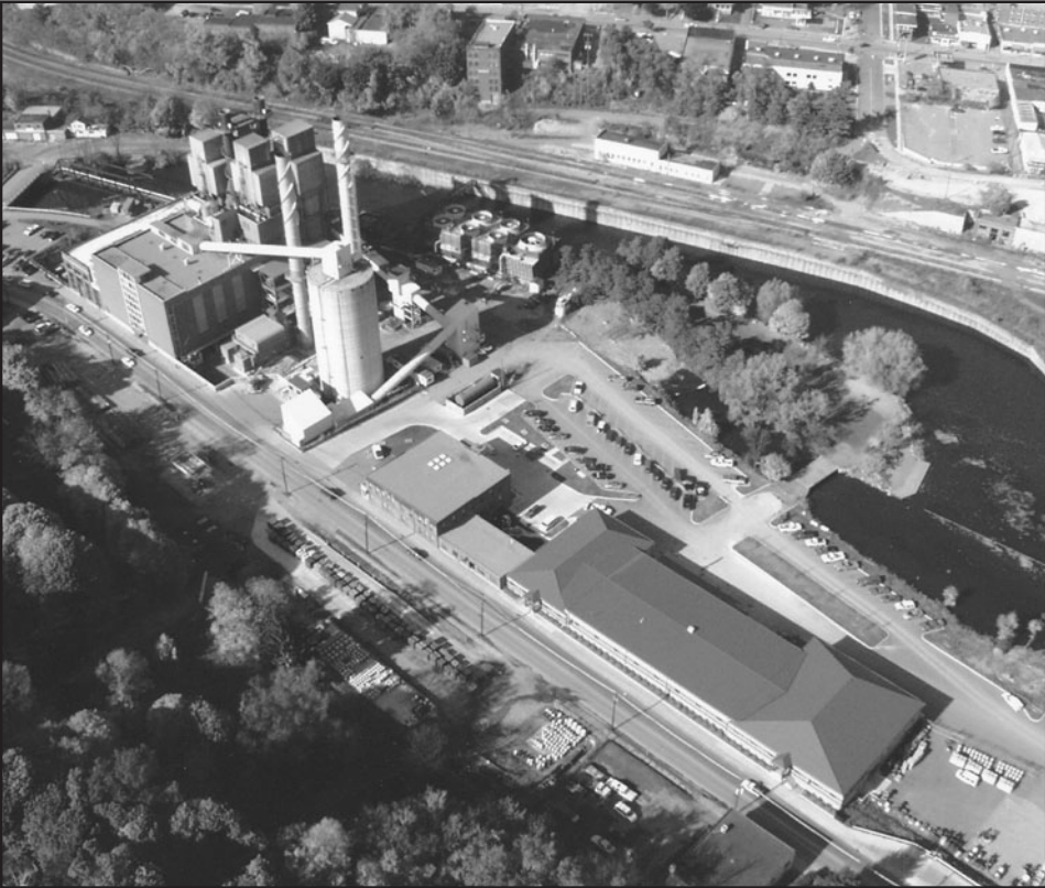
The Board of Public Utilities' Samuel A. Carlson Electric Generating Station, Business Offices and Line Department Garage.
